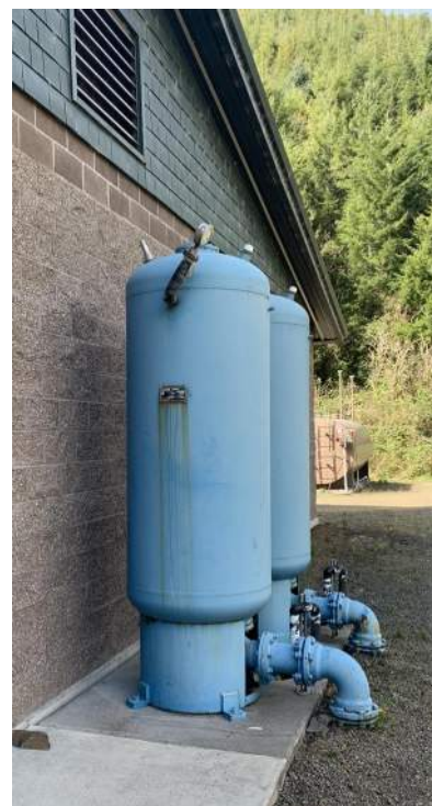
Photograph 2-6. Horn Creek Hydropneumatic Tanks
