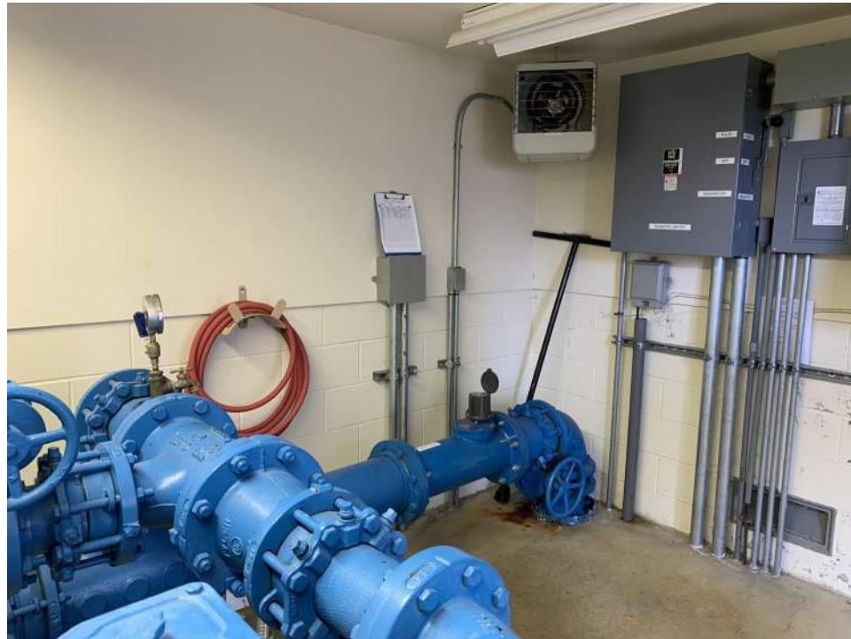
Photograph 2-16. 300K Booster Pump Piping
