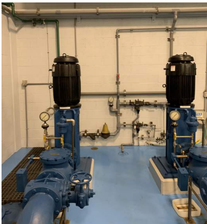
Photograph 2-5. Horn Creek Finished Water Pumps
