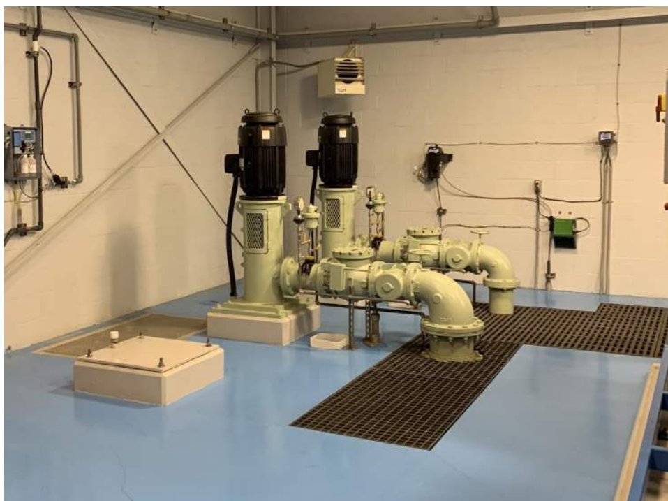
Photograph 2-3. Horn Creek Raw Water Pumps
