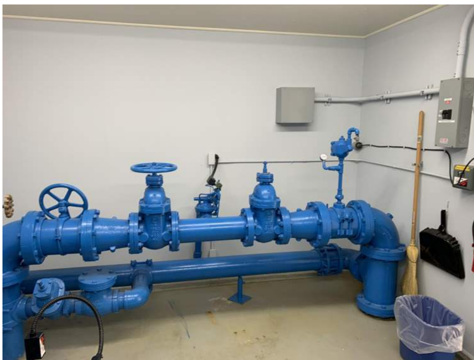
Photograph 2-13. 100K Booster Pump Piping
