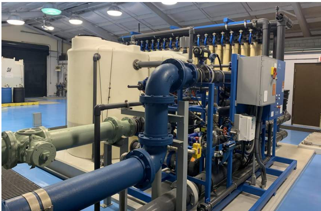
Photograph 2-4. Horn Creek Microfiltration System
