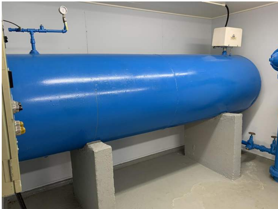
Photograph 2-11. 100K Hydropneumatic Tank
