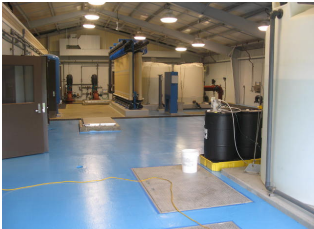
The Horn Creek Process Room
