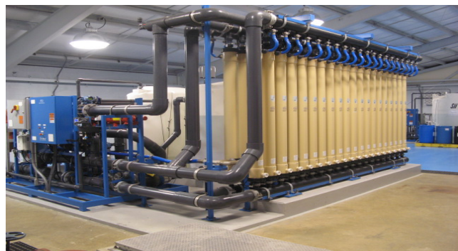
Horn Creek Micro-Filtration Membrane Modules. Each Module Contains 6,500 Membrane Fibers!
