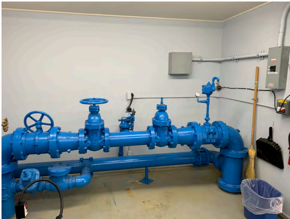
Photograph 2-13. 100K Booster Pump Piping
