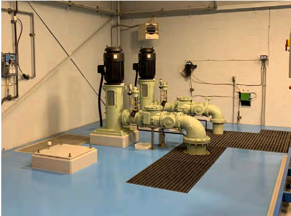
Photograph 2-3. Horn Creek Raw Water Pumps
