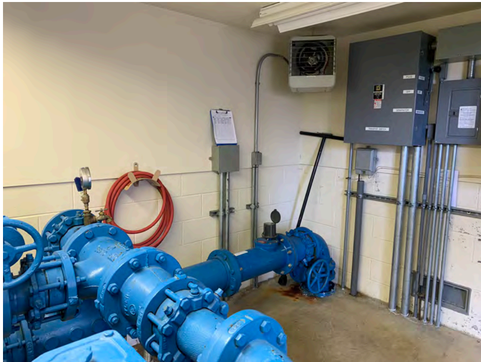
Photograph 2-16. 300K Booster Pump Piping
