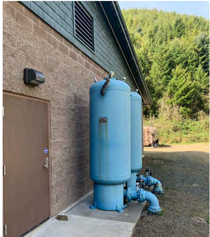
Photograph 2-6. Horn Creek Hydropneumatic Tanks
