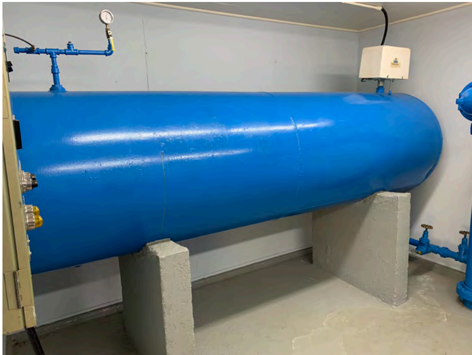
Photograph 2-11. 100K Hydropneumatic Tank
