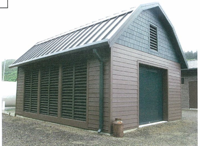
North and West Sides of the Horn Creek Generator Building. Rusted Milk Can by Spencer Hurliman. August 2011.
