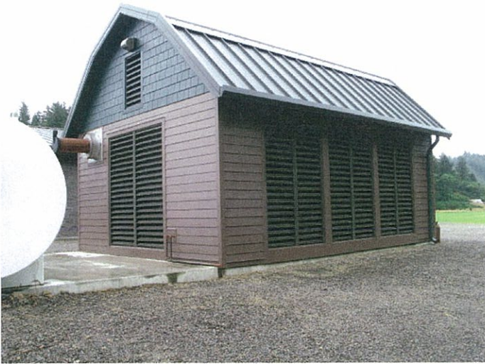
East Side of the Horn Creek Generator Building. August 2011
